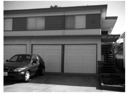
Older “soft-story” buildings with habitable space above garages are some of the more vulnerable building types in the event of an earthquake.
